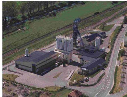
Figure 1. Backfilling plant in Sondershausen
