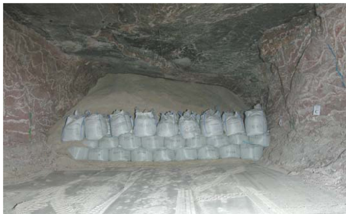
Figure 3: Backfilling of a mining site with big bags
