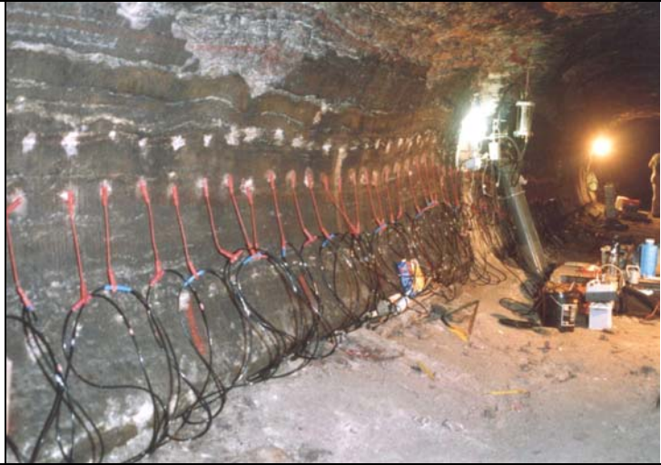
Figure 1: Injection test site during the geoelectrical measurement.
