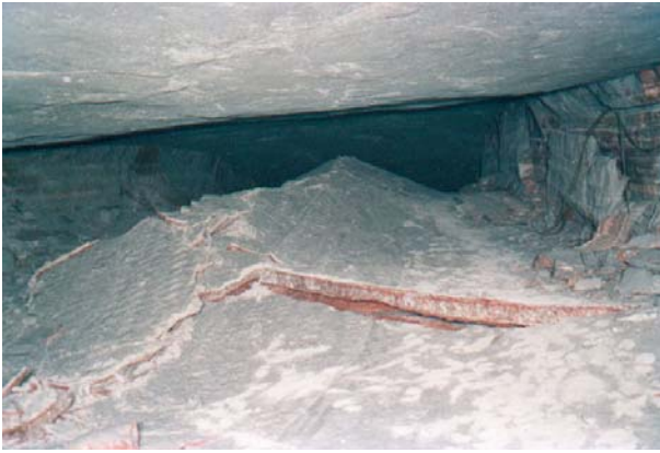
Figure 2. press-ups of the drive way due to high formation pressure.
