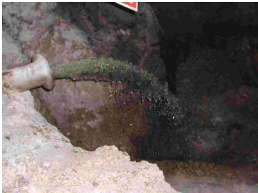
Figure 2. Mining site backfilled by hydraulic backfilling - end of pipe –
