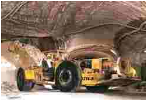
Figure 5. Backfilling of a mining site with bulk goods
