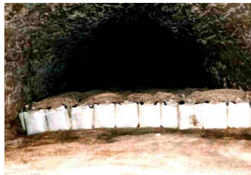
Figure 4. Backfilling of a mining site with big bags
