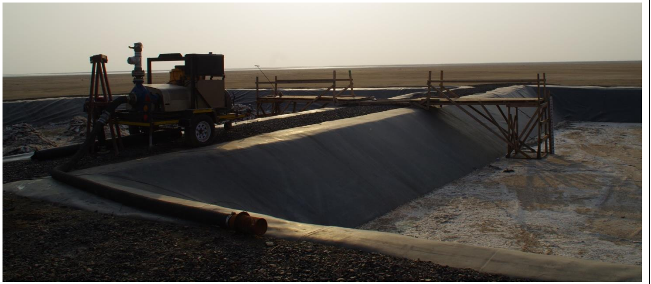
Picture 4: Evaporation pond with a mobile brine pump. The pond in the background is harvested and the pond in the fore ground is ready for filling.
